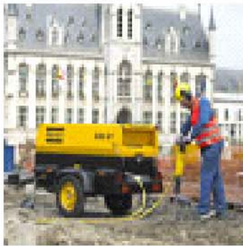
Compressors and Generators
